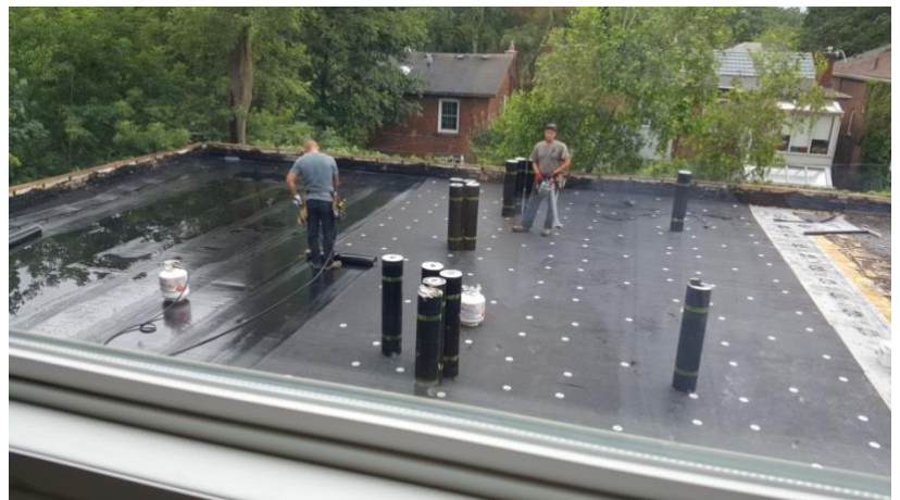
Above: Roofing crew installing new gym roof in July
